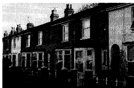
Victorian Terrace, Greenhill Road
