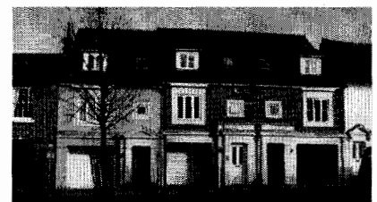
Modern Infill – Broad Street
