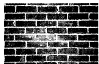
Lime Mortar Repointing
