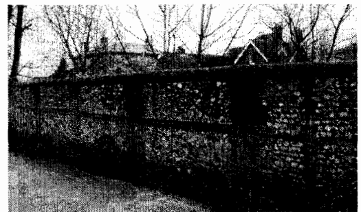
An original wall
