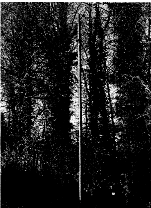
The 'Orange' phone mast
