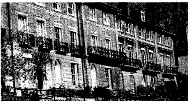
Clifton Terrace - the first development
