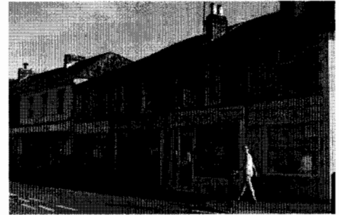
Stockbridge Road shops
